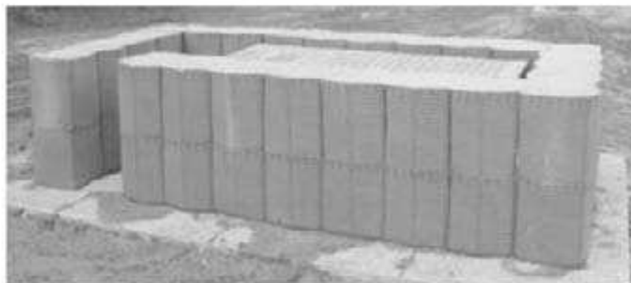
Second layer in place and filled
