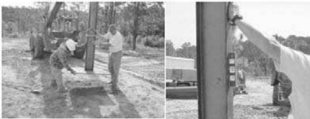
Figure 8-77. Positioning and installing columns.
