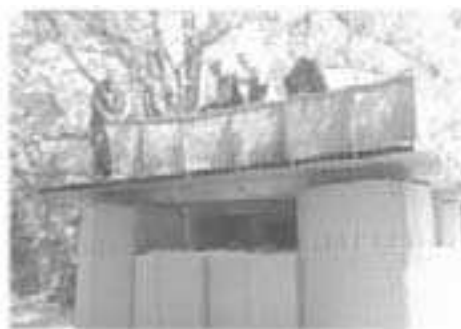
Placing Concrete container around roof perimeter
