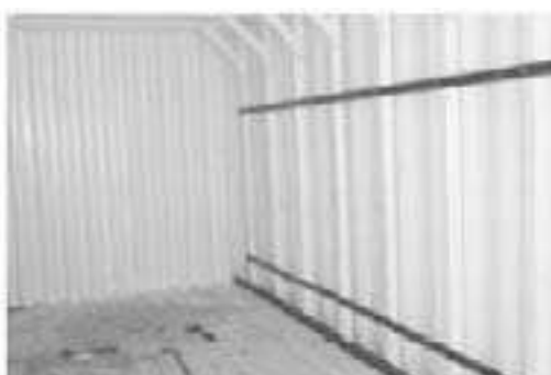
Flat bar straps attached to frames
