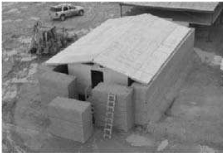
Figure 8-35. SEAhut Retrofit for Overhead Protection
