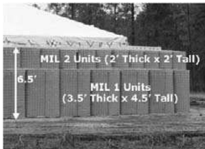
Figure 8-6. Mil 1/Mil 2 Hesco Bastion soil-filled wall
