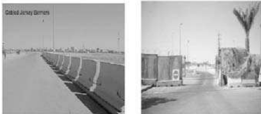
Figure 6-10. Cabled Concrete Barriers
