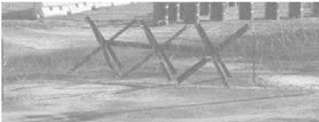
Figure 6-19. Cabled steel hedgehog
