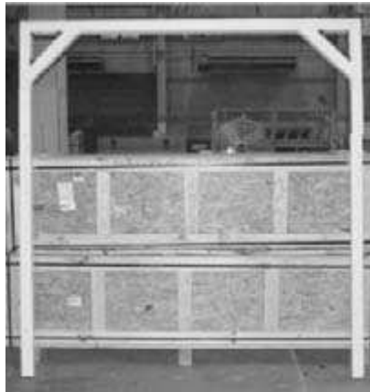
Figure 8-56. Photo of assembled steel frame section.
