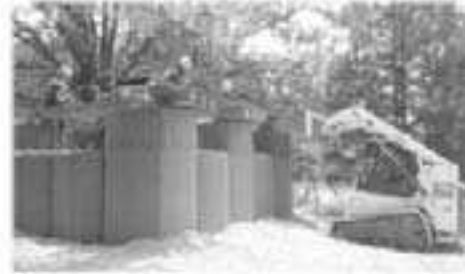
Placing Composolite panels on roof supports
