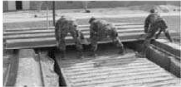
Place sheet piling roof
