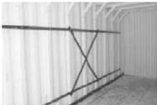
Diagonal bracing in place
