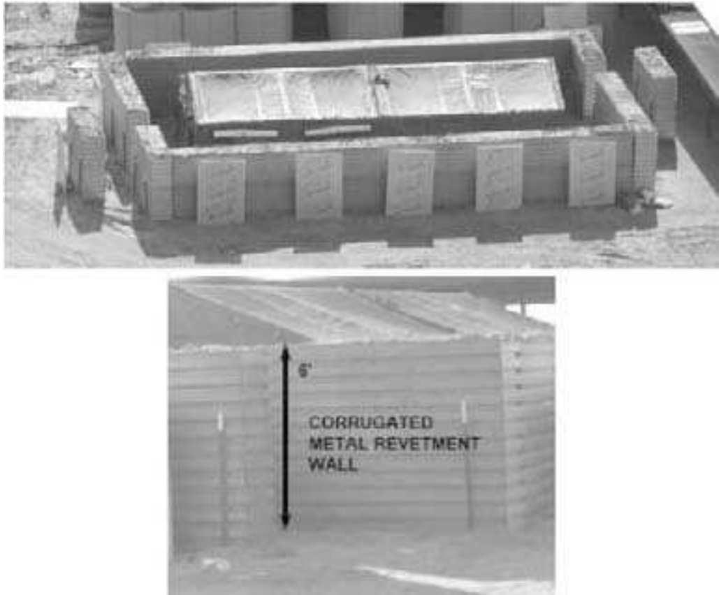
Figure 8-9. Metal bin revetment used for sidewall protection
