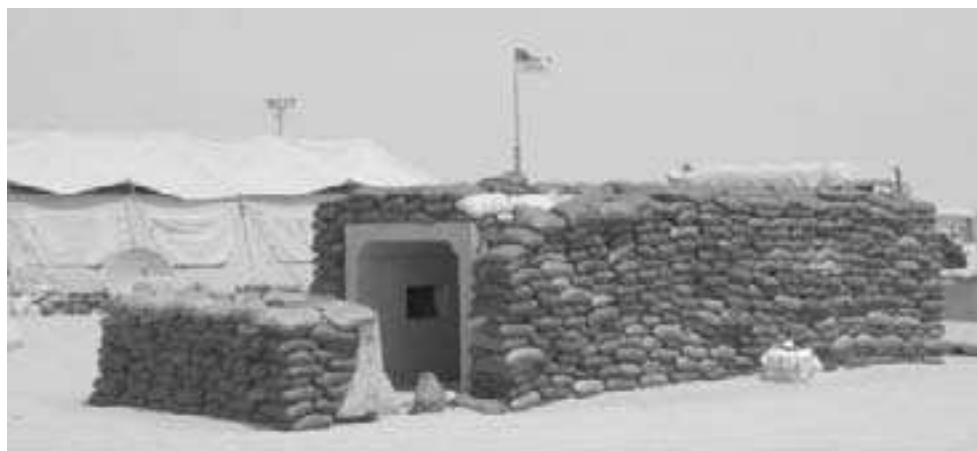
Figure 8-36. Improvised Bunker using Concrete Culvert Sections.
