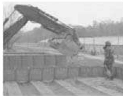
Fill Concertainer and center of roof
