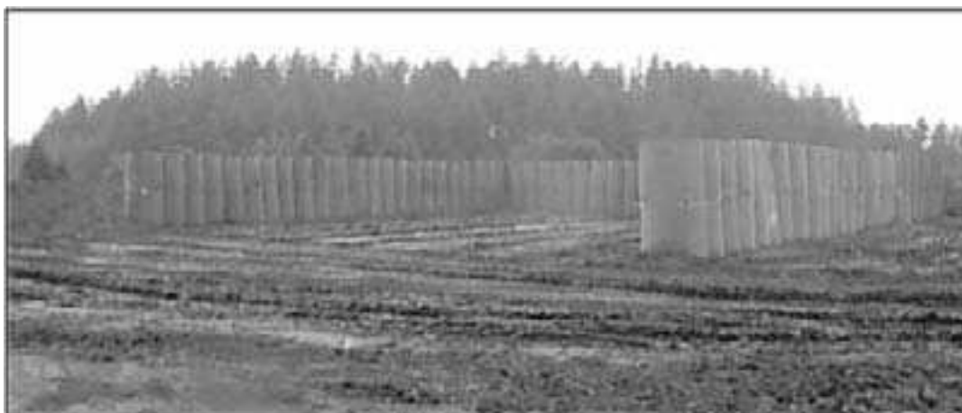
Figure 8-17. Hesco revetment design for helicopter protection
