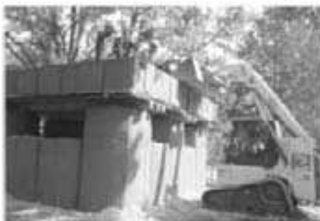
Placing soil cover on top of bunker
