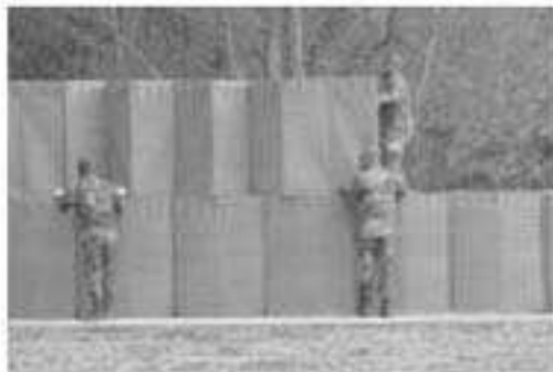
Placing second layer
