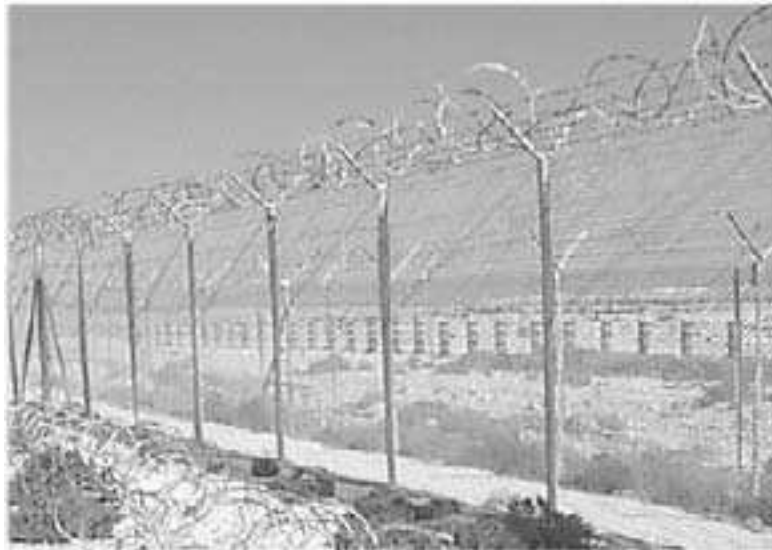
Figure 6-2. Metal mesh fence with razor wire and barbed wire outriggers
