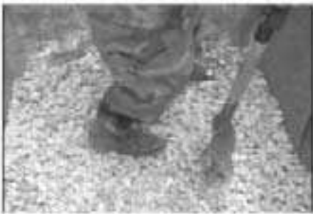
Compact fill into the sides and corner
