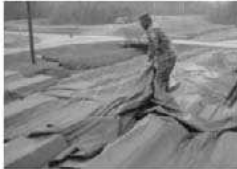
Place waterproof membrane
