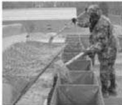
Fill Concertainer and center of roof
