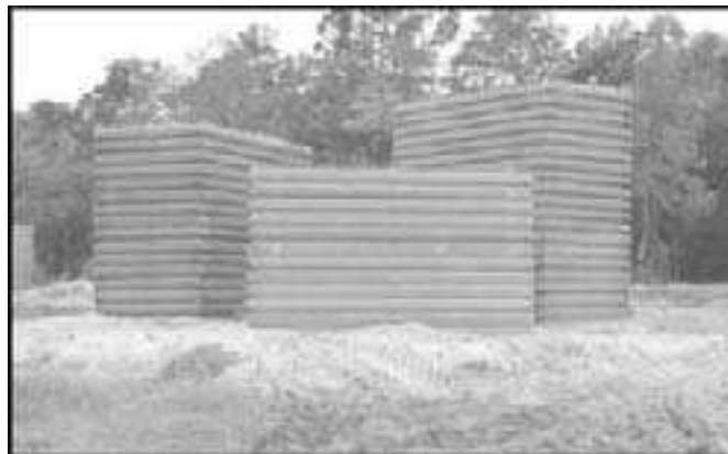
Figure 6-23. Metal revetment walls
