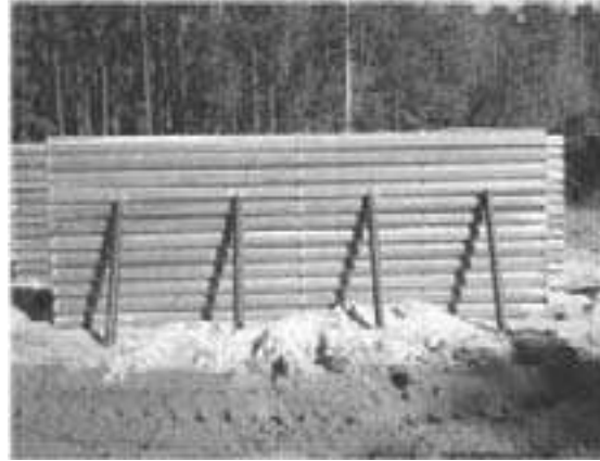
Figure 8-10. Bracing of walls for near miss 122mm rocket threat
