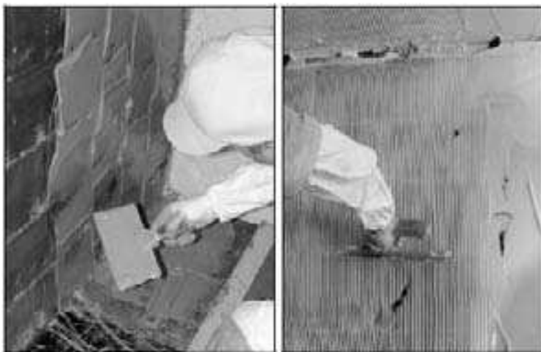
Figure 8-94. Trowel-on polymer retrofit system
