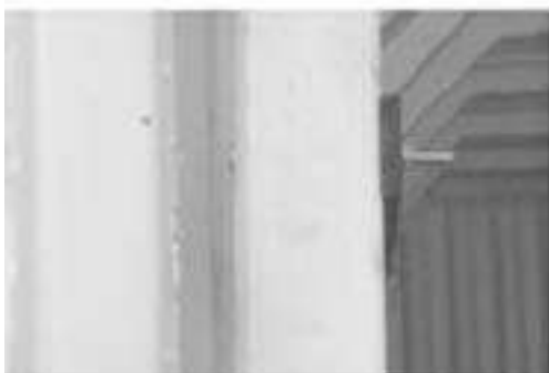
Flat bar connected to frame with bolt; Note head of bolt is on outside of frame
