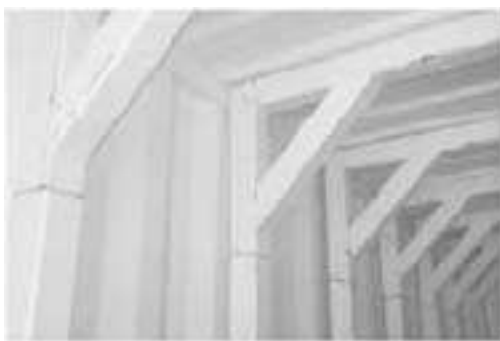
Frames installed at 2' o.c.
