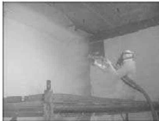
Figure 8-93. Spray-on polymer retrofit system
