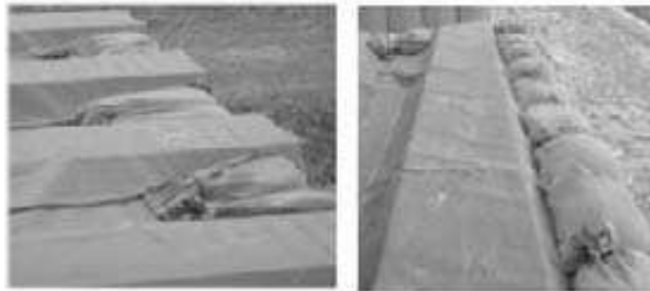
Sand bags used to level perimeter of roof
