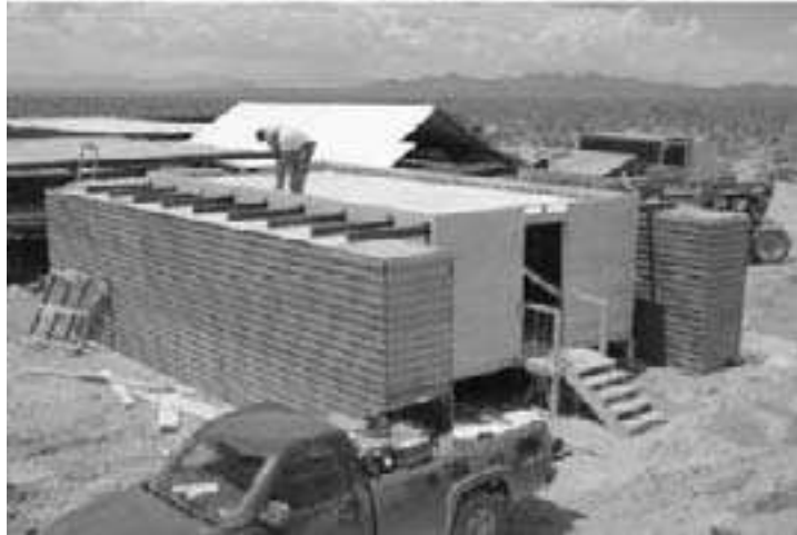
Figure 8-34. Placing Shielding Layer in SEAhut Retrofit
