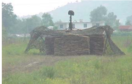
Figure 3.13. Sandbags Used for Fragment Protection
