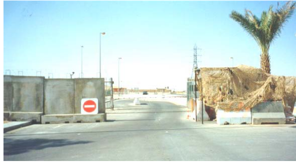
Figure 3.12. Bitburg Barriers Employed for Counter-mobility
