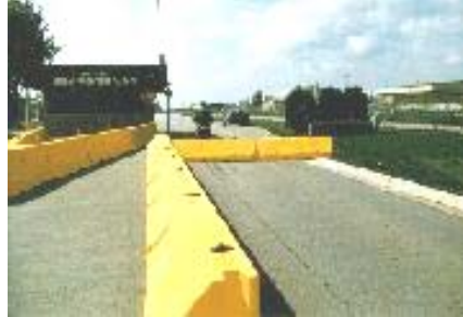
Figure 3.14. Water Filled Barriers Used for Counter-mobility
