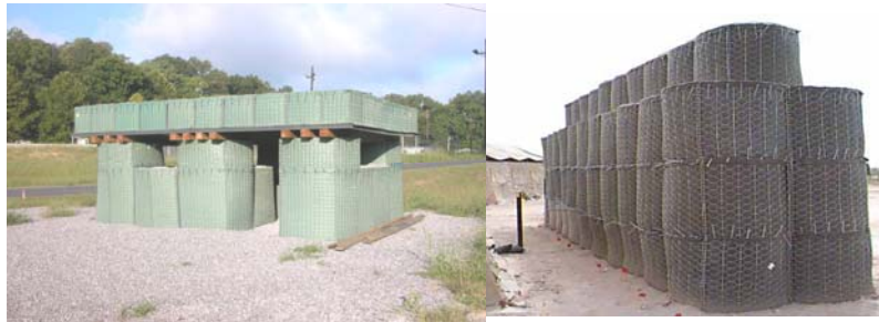
Figure 3.15. Concertainer Styled Barriers Used as Blast Walls and Fighting Positions (Concertainer Construction Techniques per ERDC Guidance)
