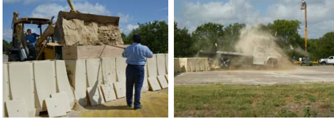
Figure A4.20. Sand-filled Plastic Barriers
