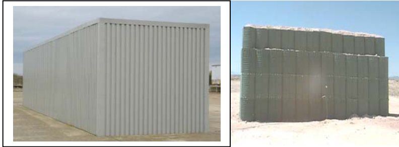
Figure 3.9. Earth Filled Barrier
