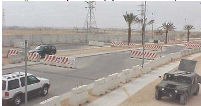
Figure 3.11. Jersey Barriers Employed for Counter-mobility
