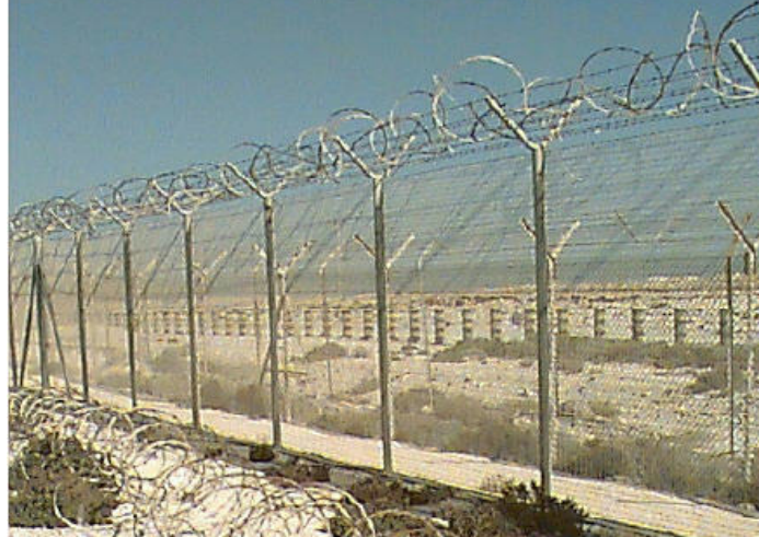
Figure 2 - Metal mesh fence with razor wire and barbed wire outriggers
